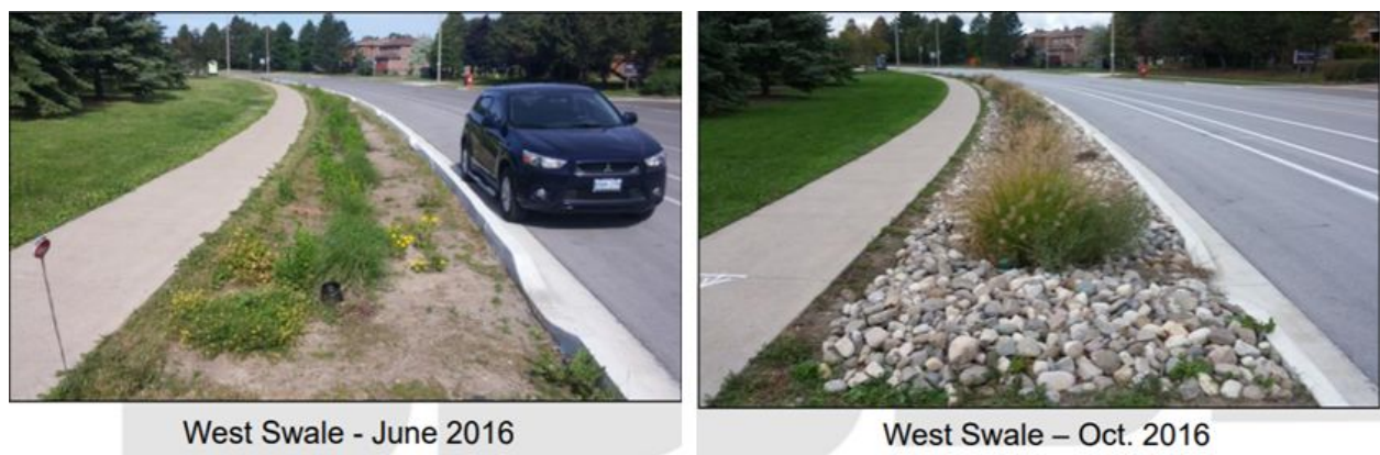
Figure 4. Biofilter swales in Brampton
