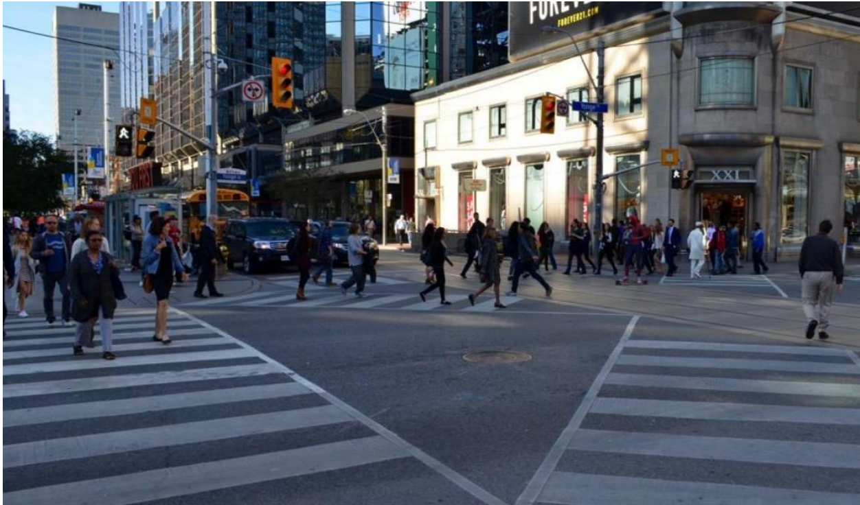
Figure 3: Pedestrian “Scramble” Crossing (City of Toronto, 2017)
